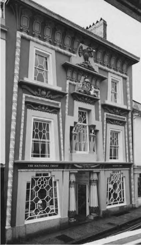
Plate 156 Egyptian House in Chapel Street, Penzance, Cornwall, of c.1835. Note the remarkable pattern of glazing-bars, the zig-zag pattern all over the torus mouldings, and the stepped corbelled arches derived from Piranesi's DM. Could Foulston and/or Wightwick have been involved? (The National Trust).
